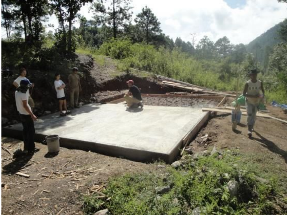
A flat and stable foundation for a Slow Sand Filter
